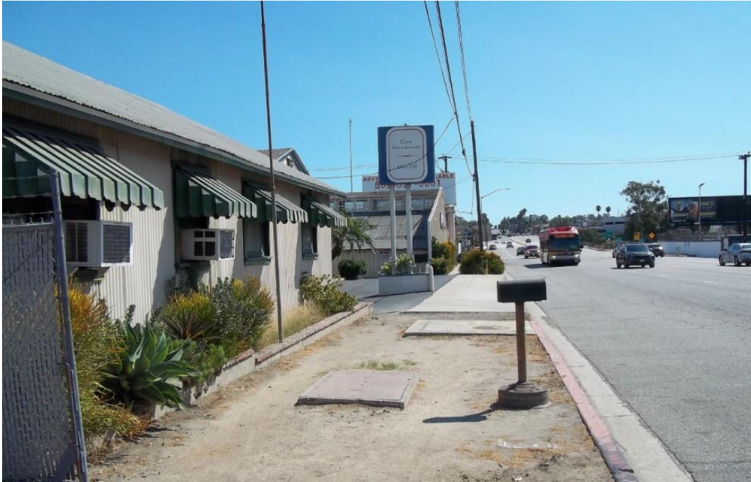
New ADA-Compliant Sidewalk
