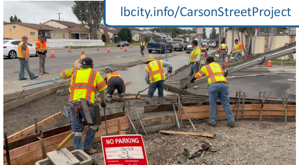
N.E. Corner of Gardenia Avenue and Carson Street
