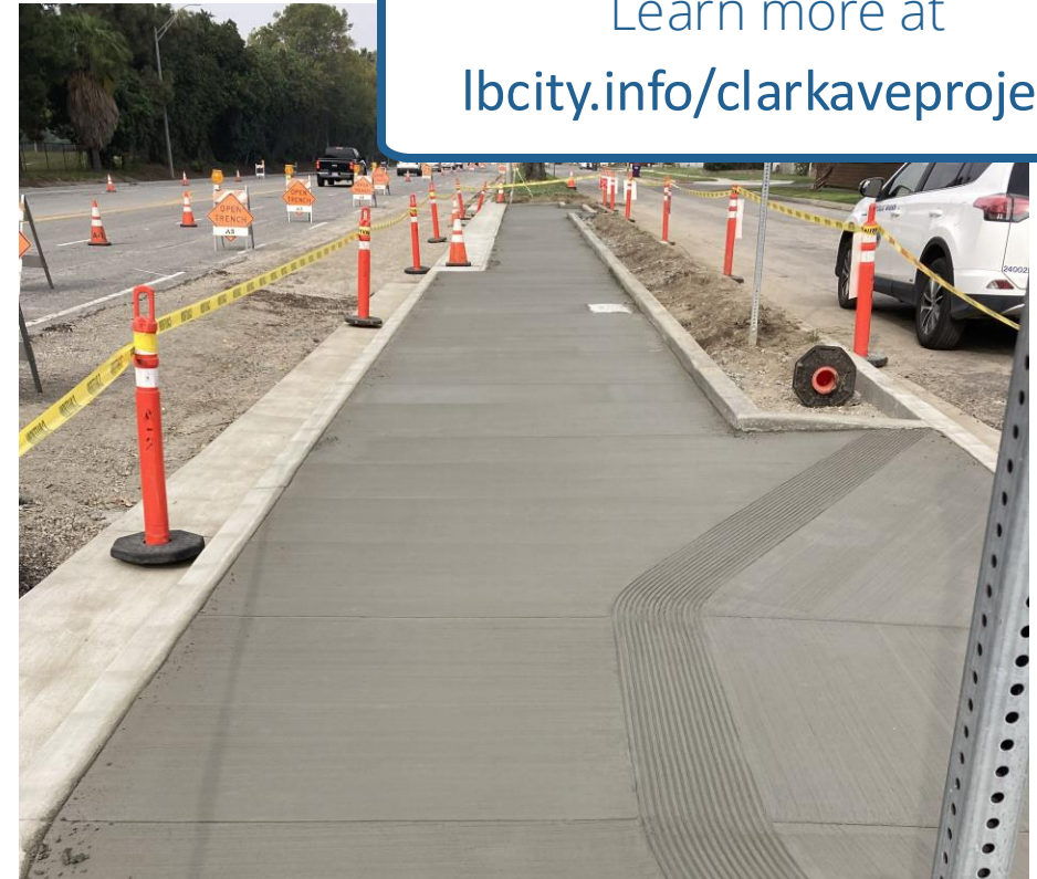
Bus Stop at Northbound Clark Ave. at Mezzanine Way
