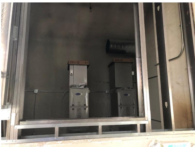
Air handlers - these are a couple of the units that will be providing heating and air conditioning to the Seminary. They are located in the front of the room on the second floor (where I believe some of the old pipe organ was located)
