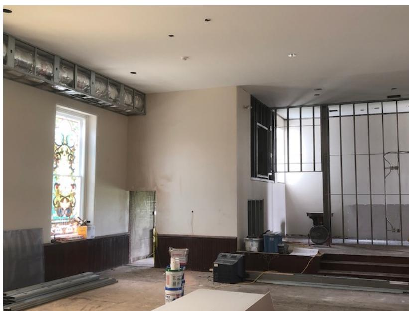
Ductwork and storage second floor - This is a picture of the new ductwork and framing to enclose it along with some of the new walls at the front of the room on the second floor.
