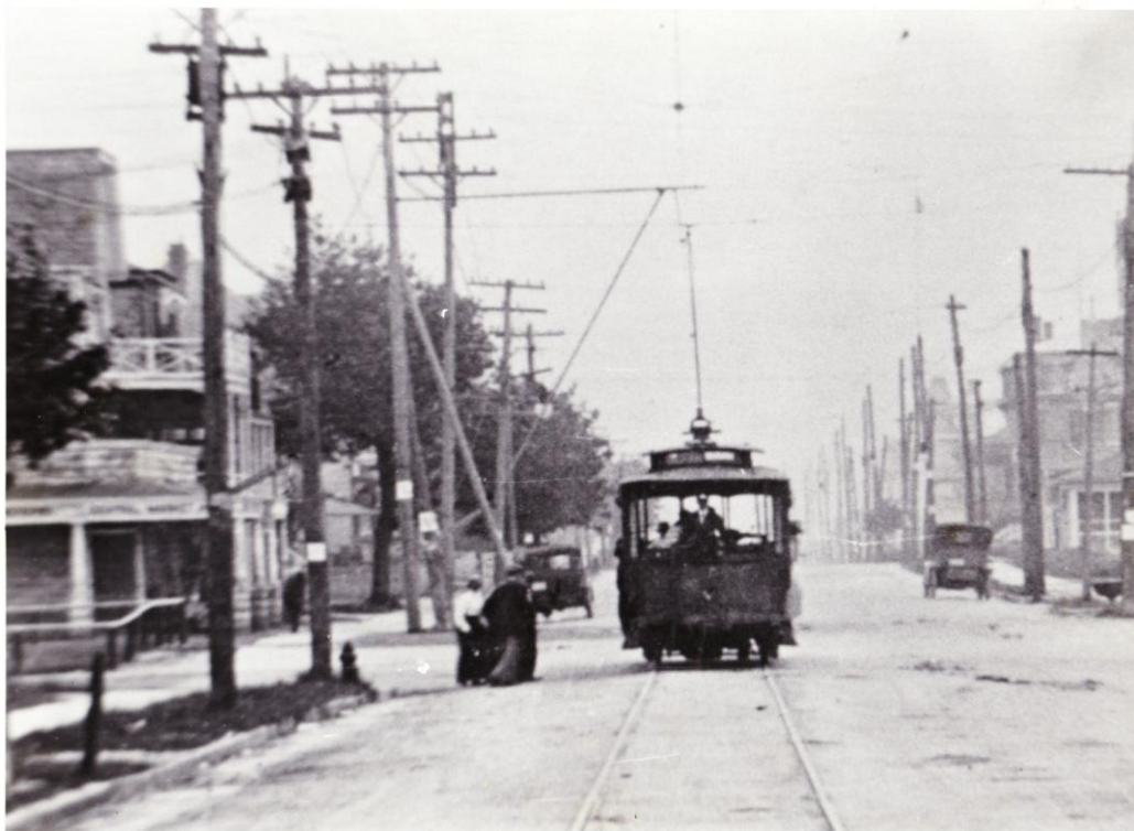
The electrified trolley on Landis Avenue, looking south...
