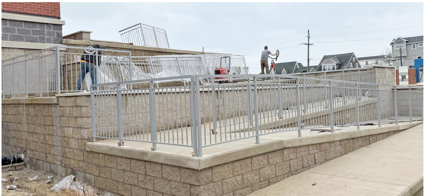
Workers are shown installing Hand Rails on the building's ADA Ramps...
