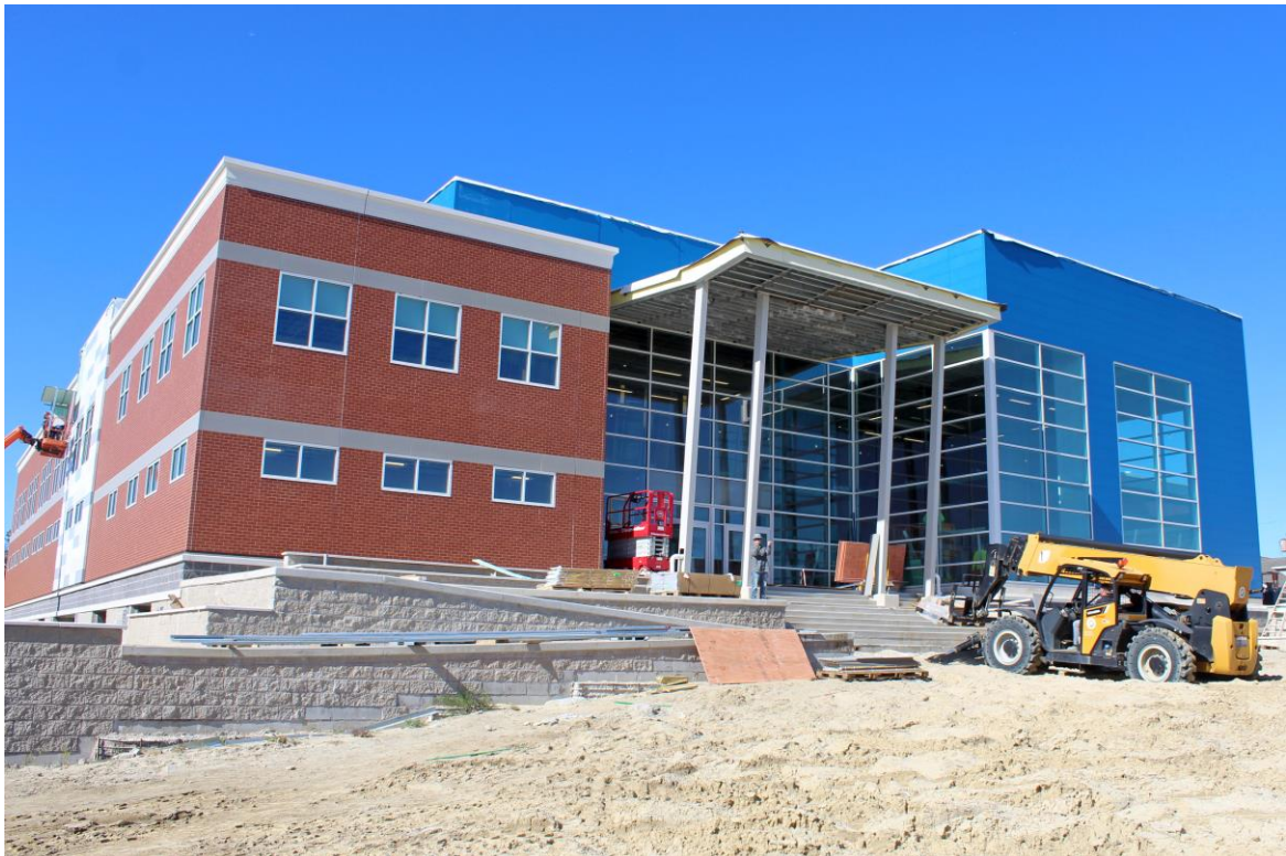
The building's main entrance (on the Central Avenue side of the property) ...
