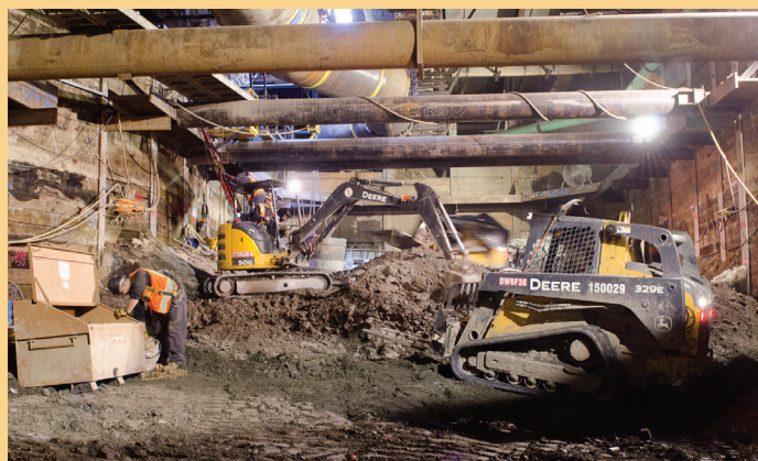
Tunnel box construction, below temporary road decking at 4th St/Flower St. Photo Credit: Ken Karagozian, 2017
