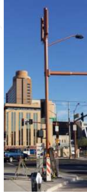
Traffic Signal Pole
