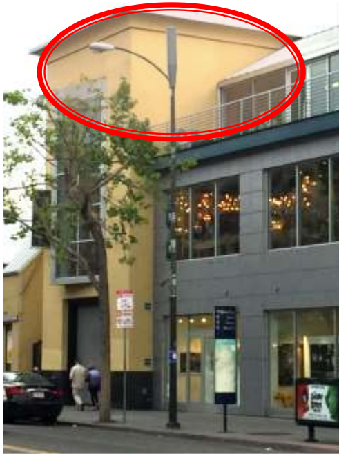
Street Light Pole
