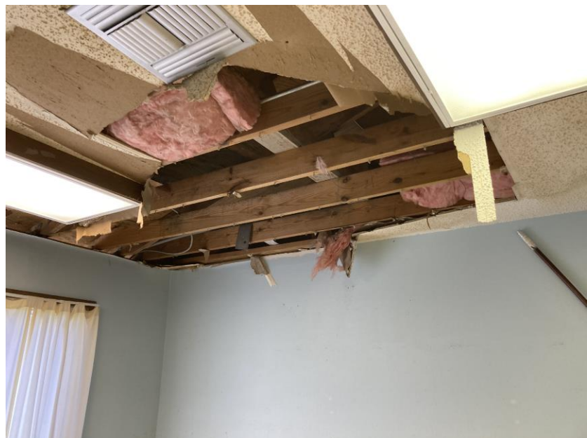
WET, MOLDY CEILINGS AND INSULATION
