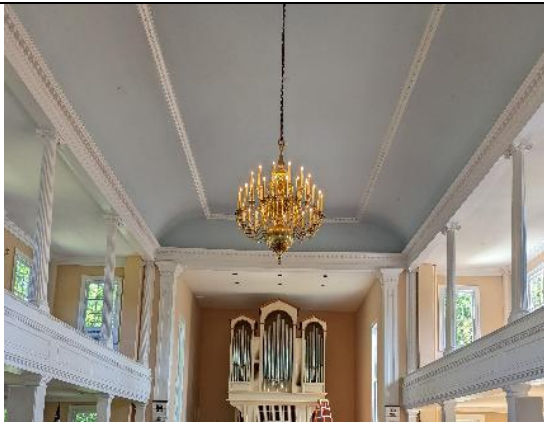
Sanctuary Chandelier – reduced wattage from 1520 watts down to 125 watts
