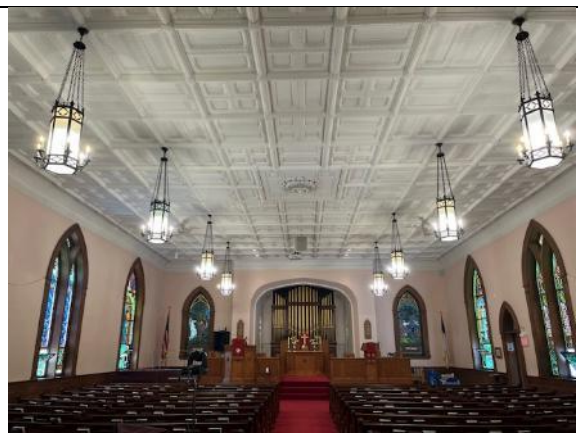
Sanctuary after – 33 watt LEDs and 17 watt FEIT Enhance candelabra bulbs at 3000K
