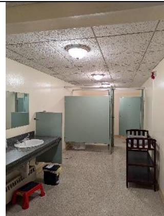
Bathroom lights – changed to 17 watt FEIT Enhance bulbs at 3000K
