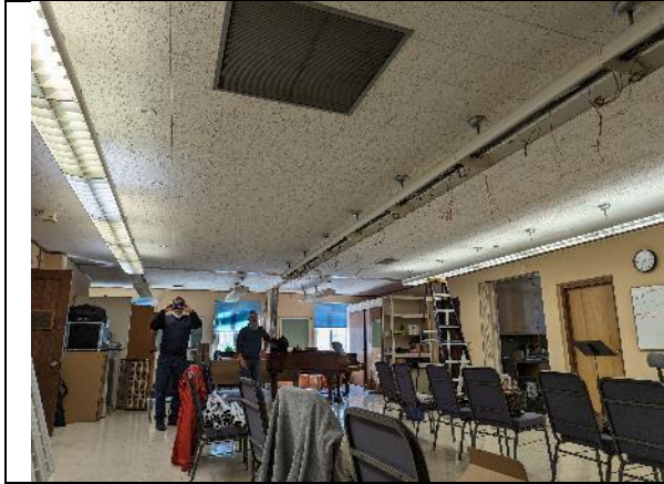
Choir Room – mid-changeover. 40 watt T12s tubes on left
