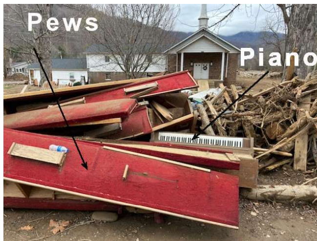
Damaged church with pews and piano in the front yard.
