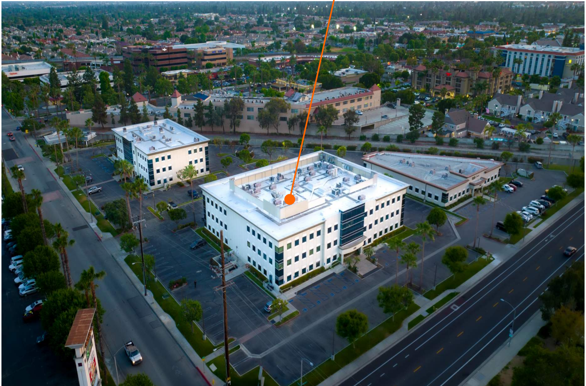
488 EAST SANTA CLARA BUILDING
