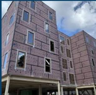
Discover how the DuPont™ ArmorWall™ System integrates five traditional building enclosure elements into a single, high-performance panel. This innovative solution offers structural sheathing, fire resistance, continuous air and water barriers, and ultra-low global warming potential (GWP) continuous insulation. By combining these features, ArmorWall™ enhances durability, efficiency, and labor savings in commercial projects. [LEARN MORE HERE](#)
