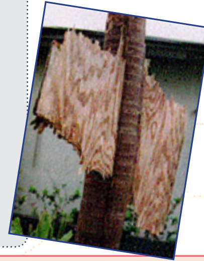
Cover photo: The roof and upper floor of this home received major wind damage from Hurricane Iniki in September 1992 (Photo: FEMA) Below: Plywood shears a palm tree during hurricane Andrew in August 1992.
