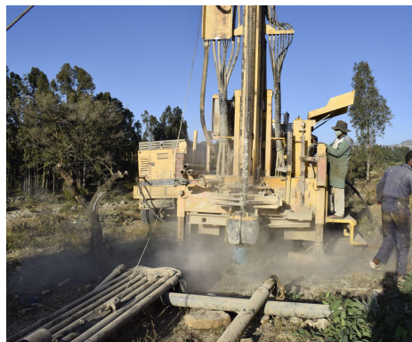
Drilling taking place.
