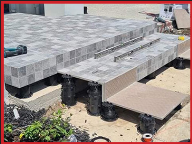
With 4" extenders available, any height can be reached to achieve your design intent on terraces, balconies, roof terraces or outdoor areas.
