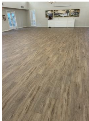
New Flooring in Malone Hall
