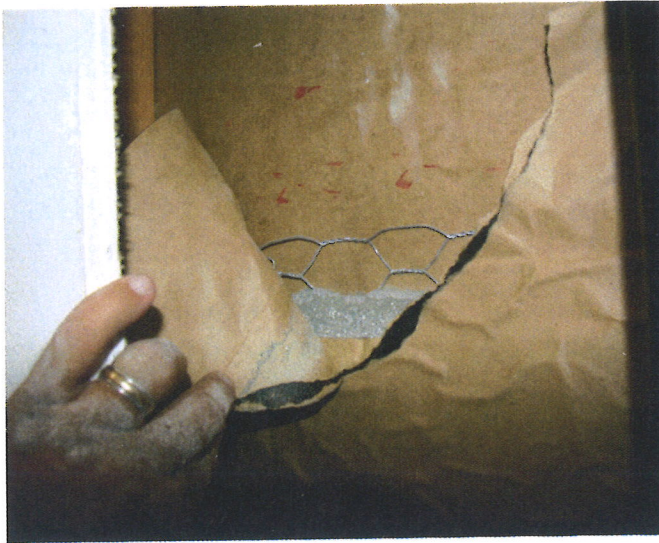
Improper scratch coat, not lapped paper-to-paper, wire-to-wire.
