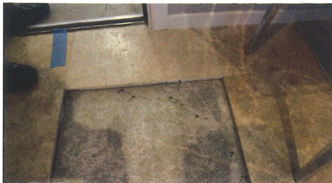
Indentation caused by concrete slab crack.
