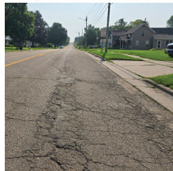
Section of Highway 89 scheduled for reconstruction.
