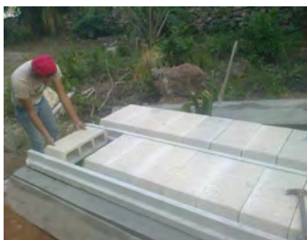
Installed septic system for toilets in Yucatan
