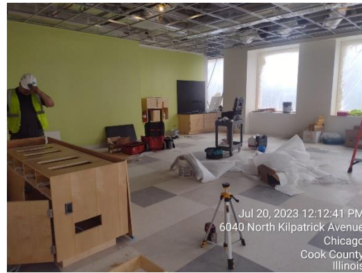
3 rd floor Classroom: Ceiling grid, flooring and casework
