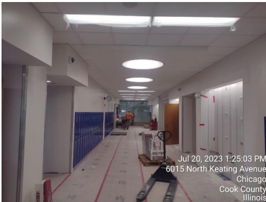
2 nd Floor Corridor: Ceiling tile and locker installation
