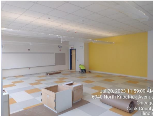
1 st floor Pre-K Classroom: Flooring and casework
