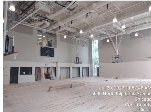
Gymnasium: Gym wood floor installation
