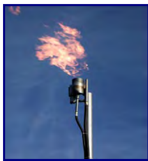
Figure 5.1.8d – Propane Burning from Flare Tower
