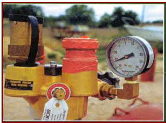
Figure 5.1.9b – New Vacuum Purged Container
