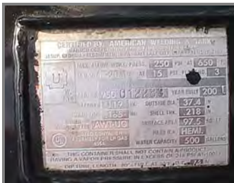
Figure 5.1.7d – Underground Tank Data Plate
