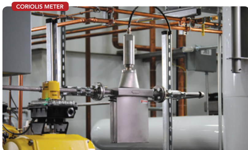
Figure 1. Such meters can directly measure mass flow with very high accuracy over a wide range of temperatures.
