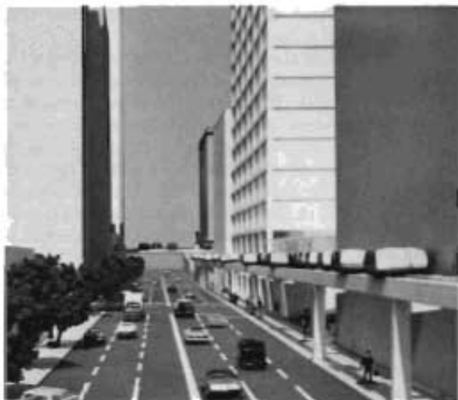
Fig. 2-5. Typical Curb-line Alignment for One-Way PRT
