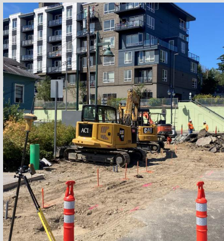
Demolition of existing pavement and sidewalk (southeast corner)
