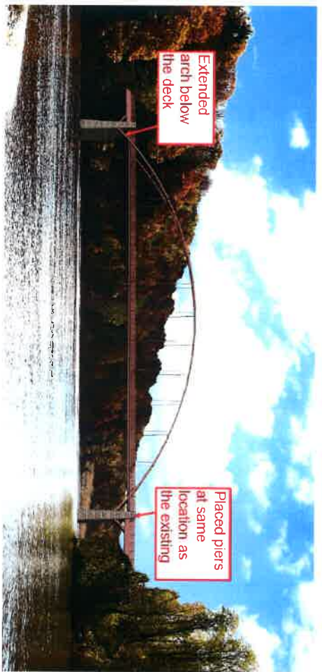
Replacement Option 3 - Tied Steel Arch
