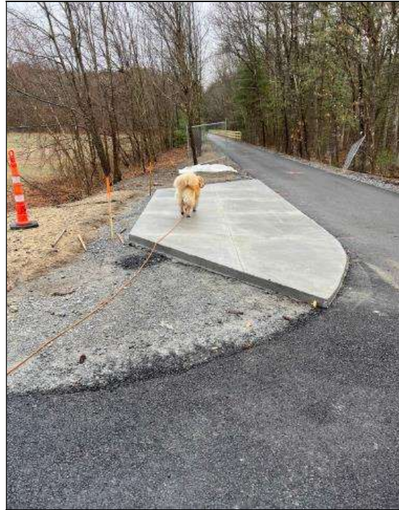
Concrete bench pad at Parkinson Field Spur
