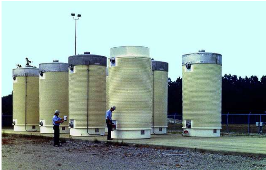
FIG. 9. TN-32 storage casks at Surrey NPP in the USA (photograph courtesy of US NRC File Photo).
