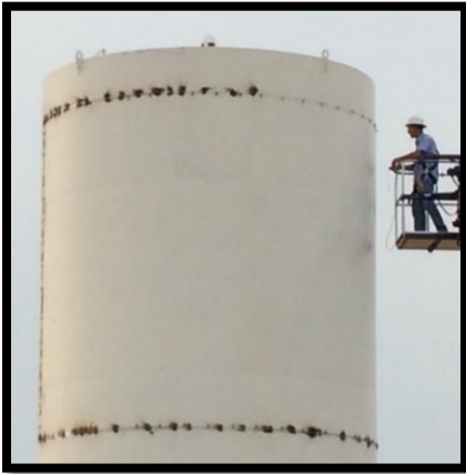
Simply mark Banner perimeter and tac-weld BannerFrameFLEX 1.5" Off Perimeter
