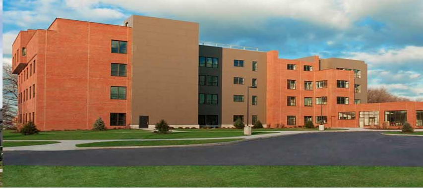
Wegman Transitional Care Center
