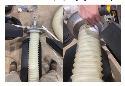
Electrician wired GridBee SN1 mixer for 220v power and installed standard 110v power cord onto the included exhaust blower fan
