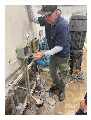
Installed hose intake support onto intake side of hose with brace using large band clamp
