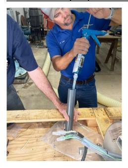
Lowered intake end of hose with support into storage tank. Set up intake end of hose at stagnant area of storage tank to encourage efficient mixing.
