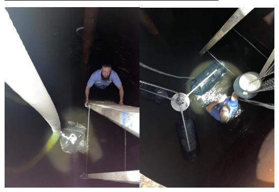
Anchored mixer securely into place using included cement anchors and stainless steel chain
