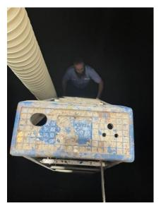
Lowered GridBee SN1 mixer into storage tank using included support chain. Placed mixer into best position available in tank to avoid spray contact with any pump intake (<u>high velocity mixer spray can damage pump intakes through friction erosion</u>)
