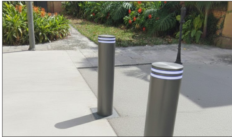
Upgraded bollards for maintenance access and clear intersections
