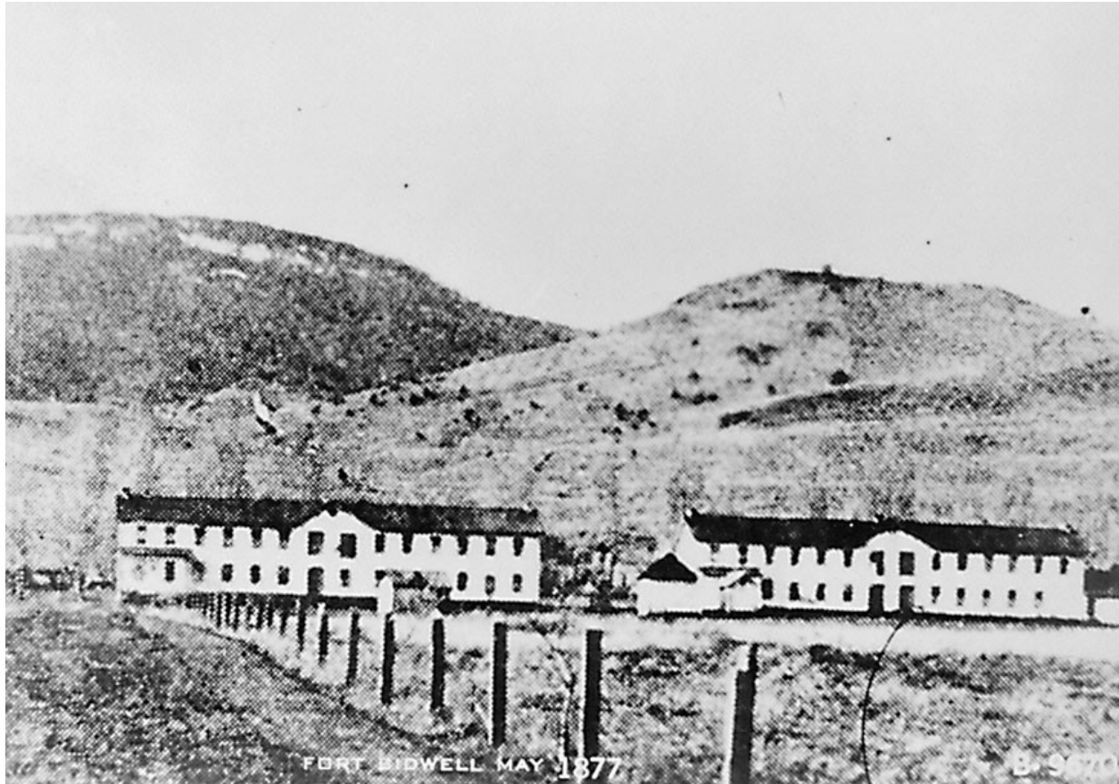
Officers' Quarters, looking west, Fort Bidwell, 1877 (Photo courtesy of the Oregon History Project) When the Fort closed in 1890, these buildings became the dormitories for the Fort Bidwell Indian School when it opened in 1898.
