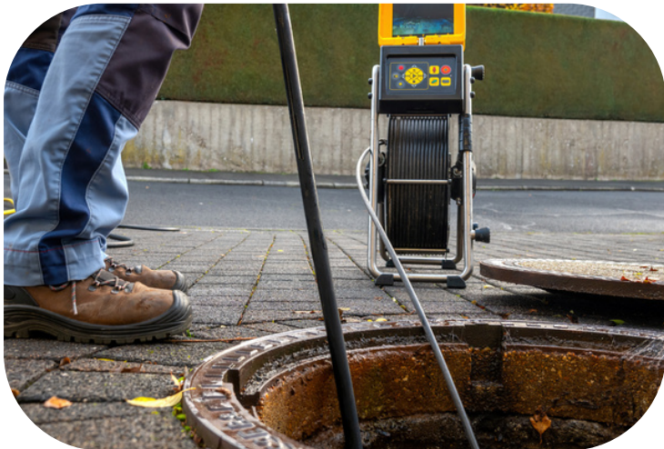
A photo of someone doing sewer maintenance
