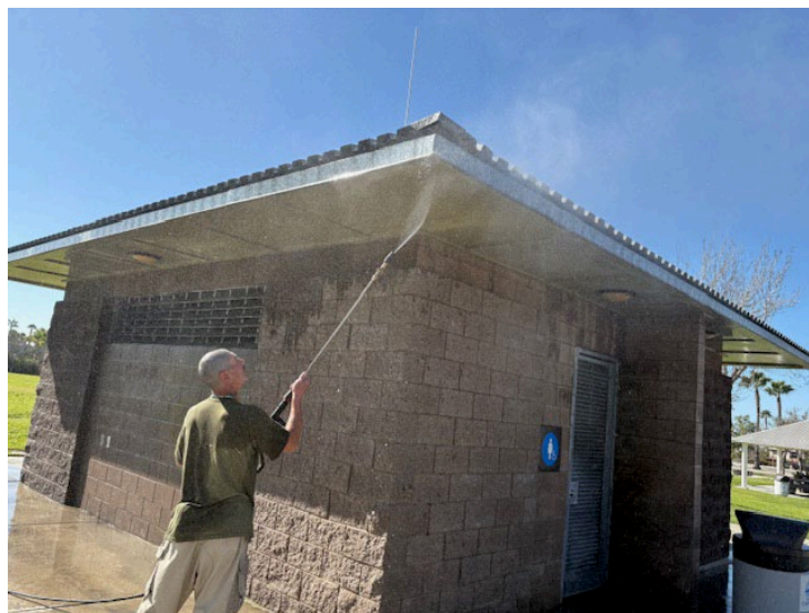
Work for Hope power washing restroom at Harvest Park.
