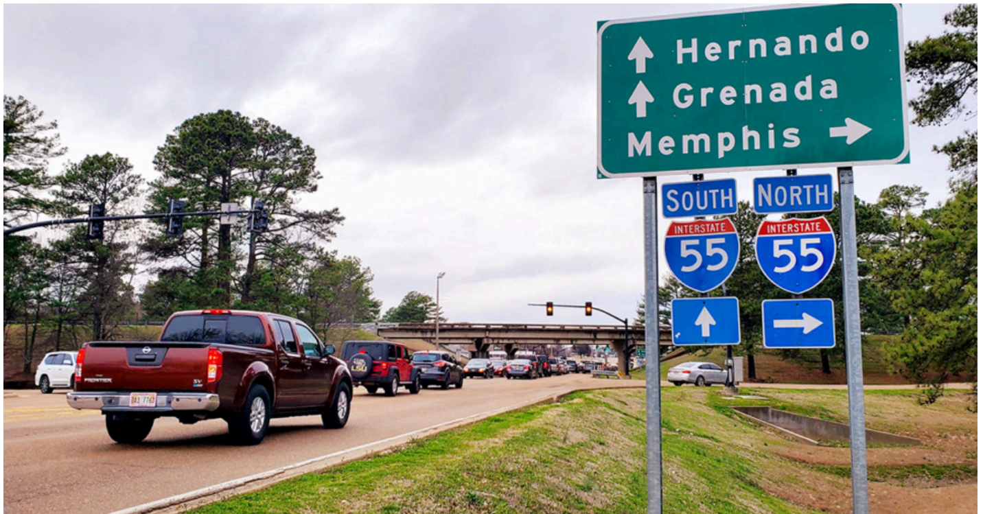
A line of traffic waits under the interstate overpass on Commerce Street in Hernando to turn north onto interstate 55. (Toni Lepascka/Special to The Daily Memphian file)
