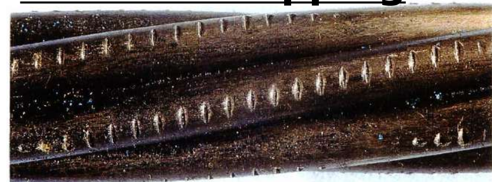
Inspection after removing epoxy coating
