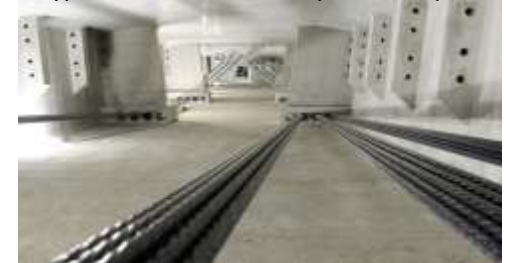
Typical External Tendon System in Japan
