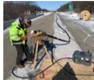
Preparation of 775 ft long tendon bundling, pulling, welding eyes and installation
