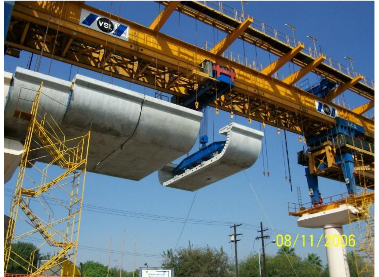
Monterrey Transit Line 2 – Monterrey, MX | MTA (Monterrey Transit Authority) | Garce Ponce Construction, VSL | Weidlinger Associates
