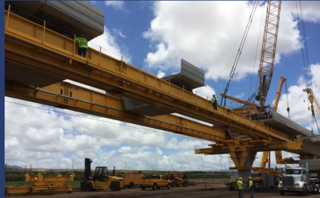
Span-by-Span Underslung Gantry
