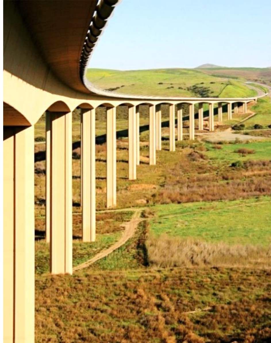
Otay River Bridge – San Diego County, CA | California Transportation Ventures | Otay River Constructors (Washington Group/Fluor) | SYSTRA IBT
