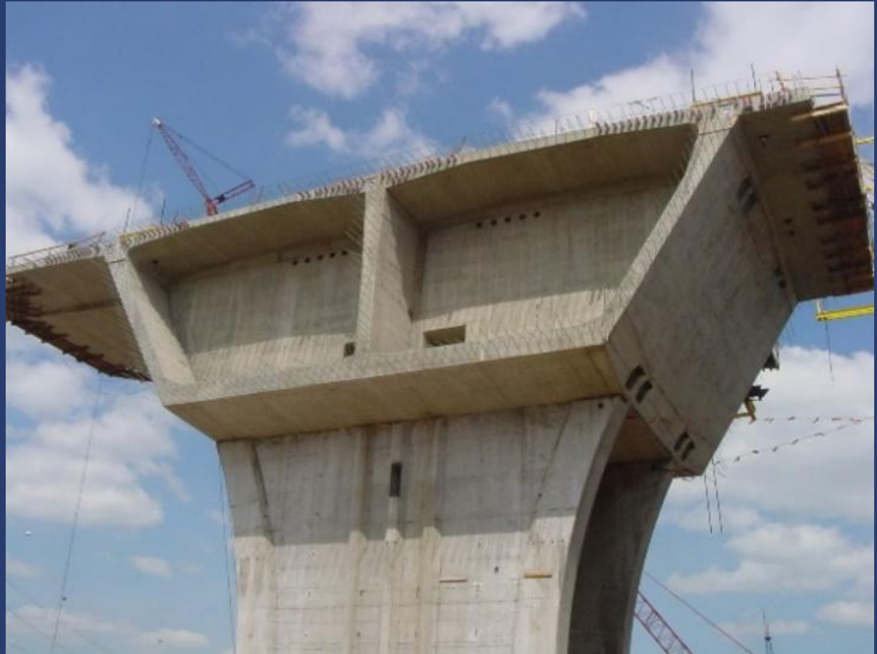
Wakota Bridge I-494 – South St. Paul over the Mississippi River | Minnesota DOT | Lunda Construction Co. | HNTB
