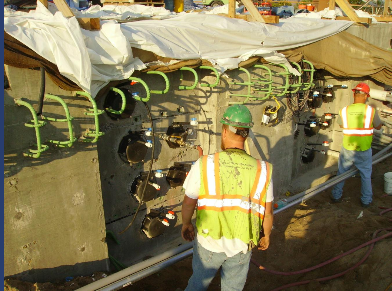
Grouting of Post-Tensioning Tendons
