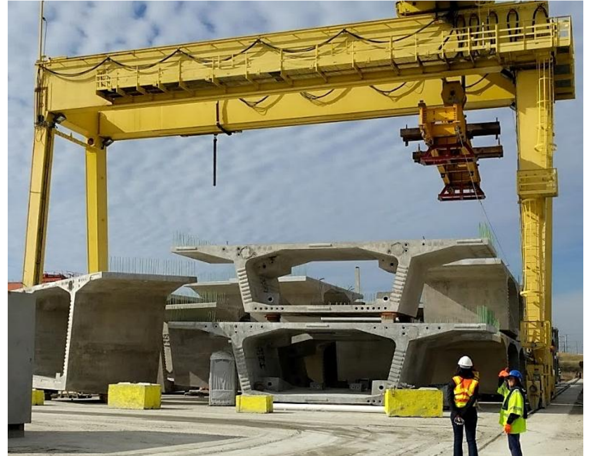
Example of Segment Stacking in Storage
