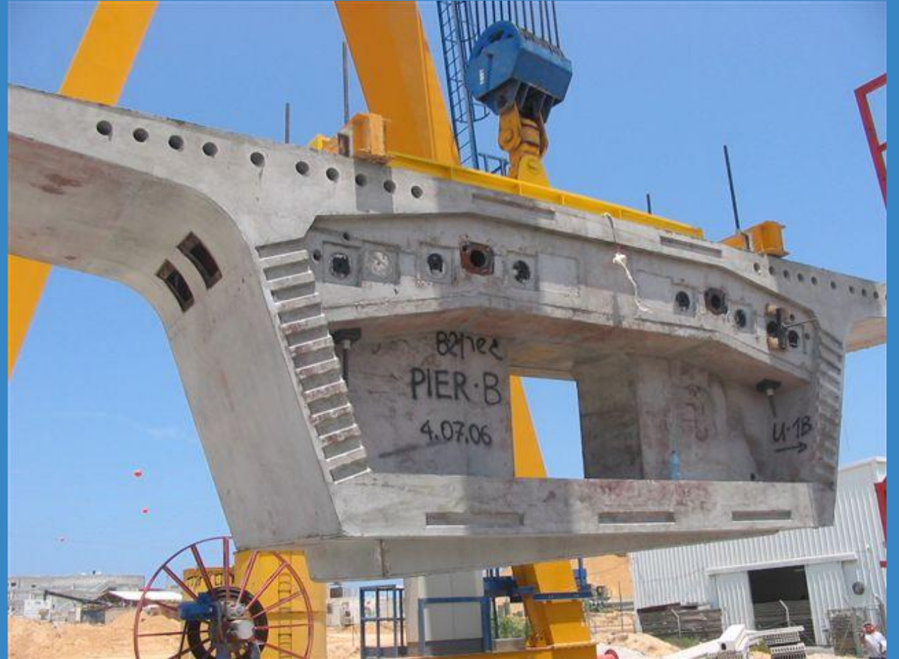
Interior Pier Segment
