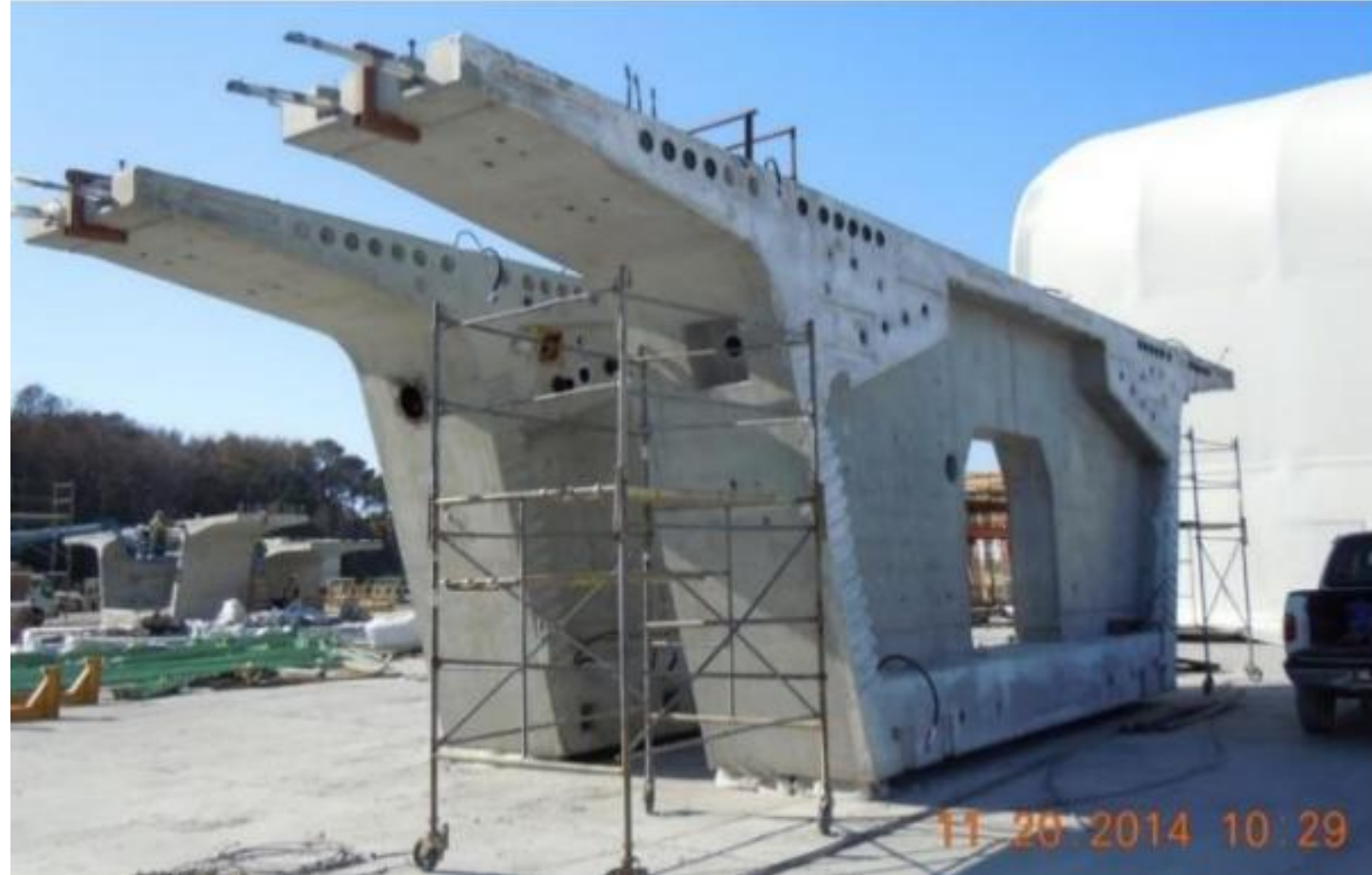
Interior Pier Segment
