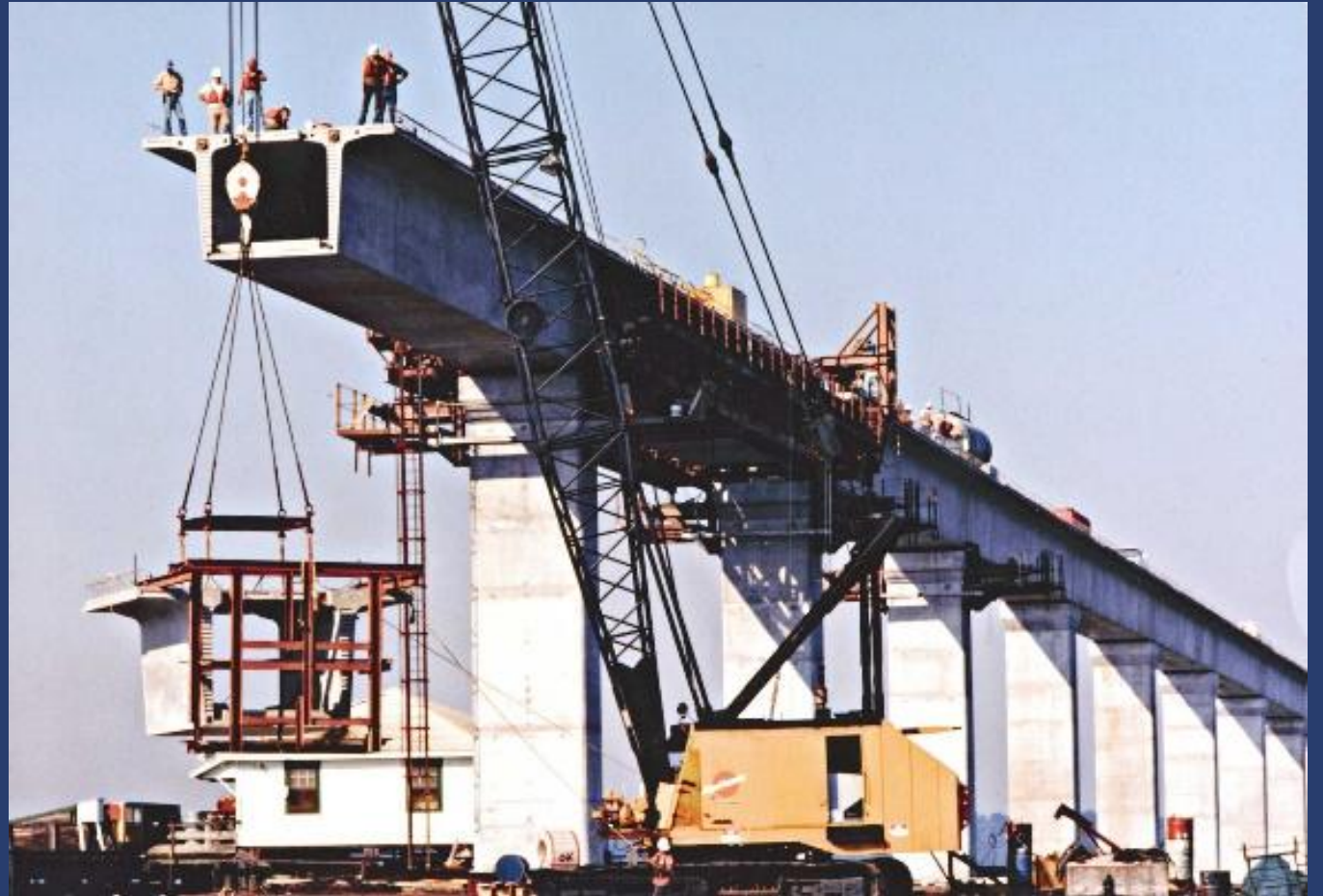
John T. Collinson Bridge – Escambia Bay, FL | CSX Railroad Figg & Muller Engineers | LoBuono Armstrong (CE)
