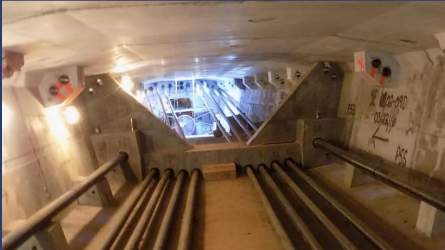
Interior View of External PT Deviating at Deviator Segment
