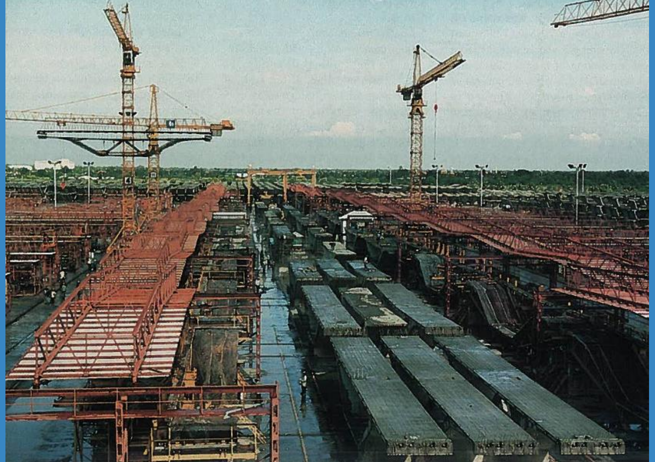
Short Line Casting Yard with over 75 Casting Machines
