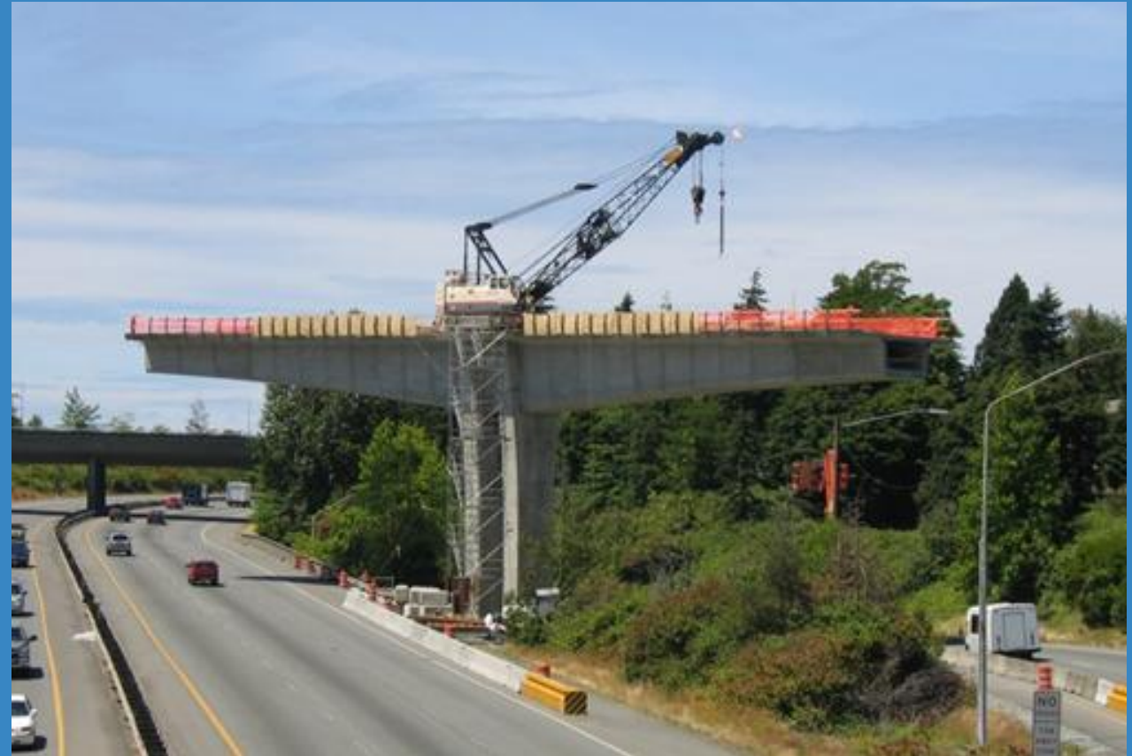
Precast Balanced Cantilever Using a Deck Mounted Crane
