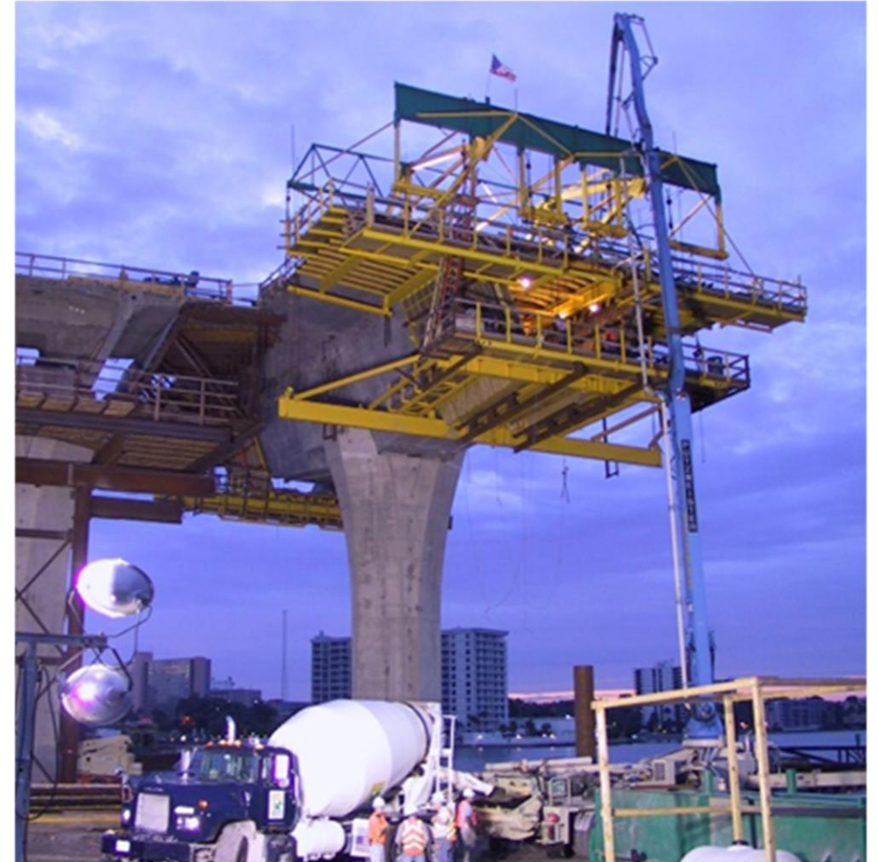
CIP Balanced Cantilever Construction
