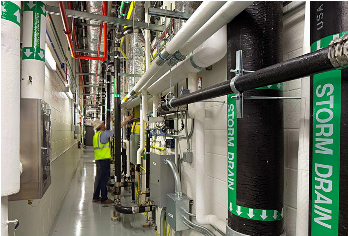
Existing WCDC Phase 2 Facilities Chase
