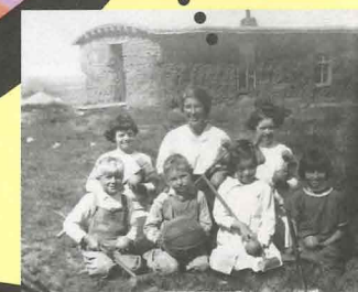
Where wood was scarce, pioneers cut sod blocks from their land to build homes and schools, like this one in Greeley County in 1910.
