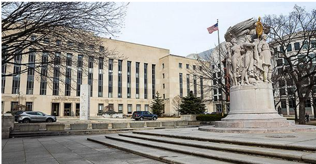
The E. Barrett Prettyman U.S. Courthouse houses the U.S. Court of Appeals for the District of Columbia Circuit. Francis Chung/E&E News
