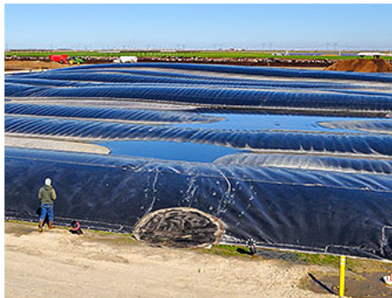
Dairy digesters the size of multiple football fields cover manure lagoons and trap methane before it's emitted to the atmosphere. Jeremy P. Jacobs/E&E News
