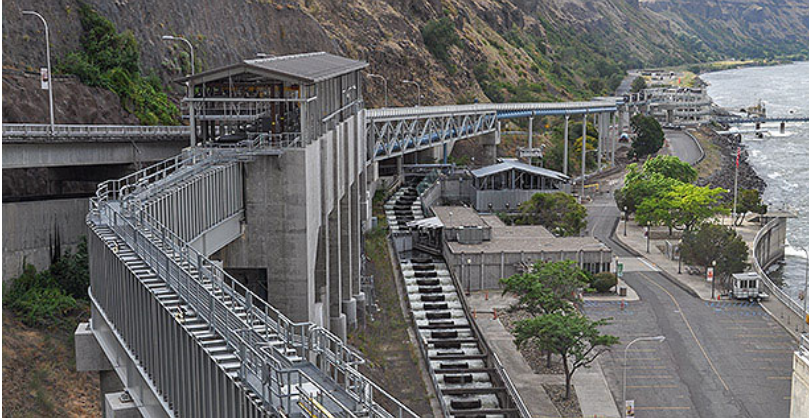
The fish ladder and other facilities at Lower Granite Dam. Jeremy P. Jacobs/E&E News
