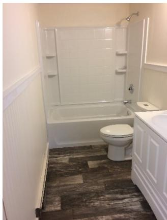
One recent project the CDP maintenance staff completed was a total bathroom renovation at one of our Harwich properties. Previously, the bathroom had a window that was located inside the shower. This led to a longstanding leak in the shower which eventually rotted the wall. Ray and Steve decided an entire remodel was needed.
