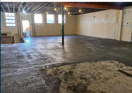
Concrete Slab Placement under Gym
