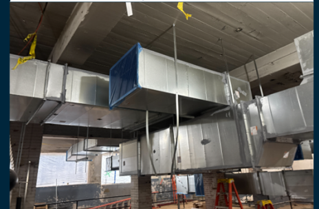
HVAC Duct Layout-Area C Level 1
