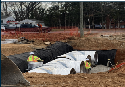
Detention Basin Install on Mohawk
