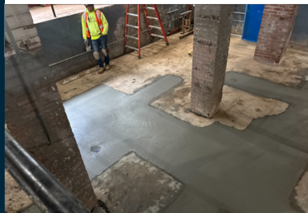
Trench Concrete Infill
