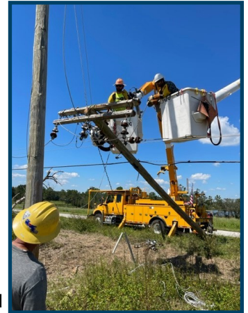
MMED employees repair a utility pole in Bartow, FL
