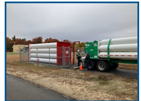
SBEC crews unload hydrogen into the hydrogen storage system
