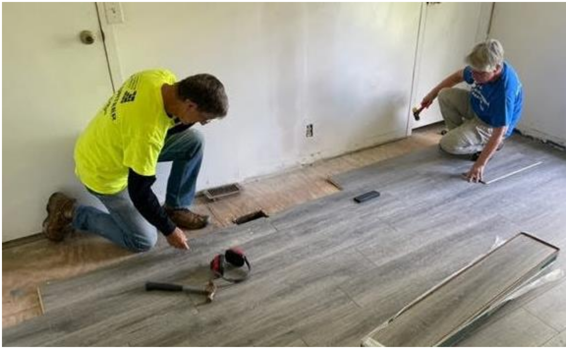
We tore up old warped flooring and put down new laminate flooring. Working on your knees is hard.
