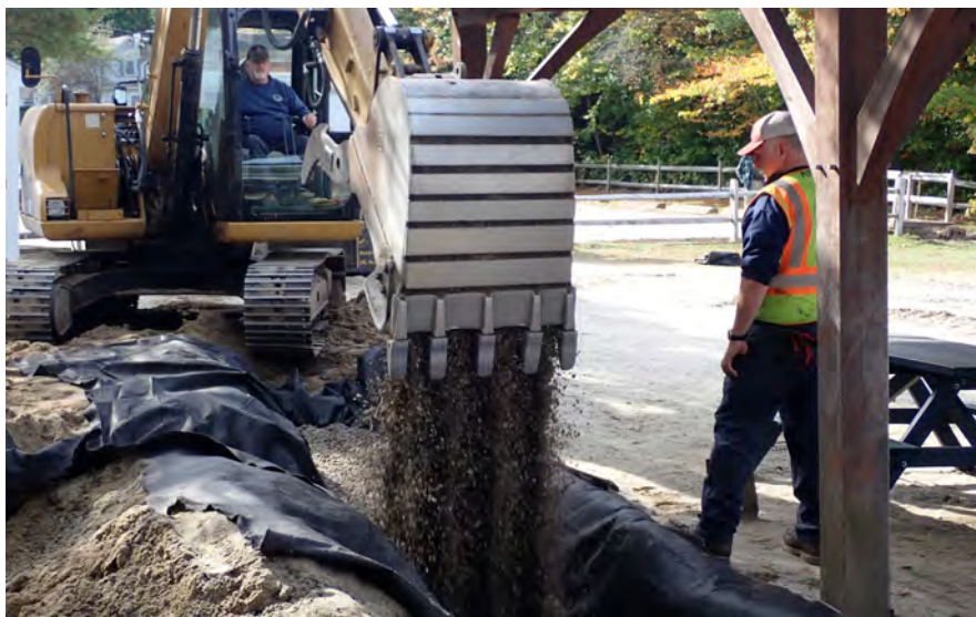
The Town of New London Department of Public Works employees constructing one of the dripline infiltration trenches.
