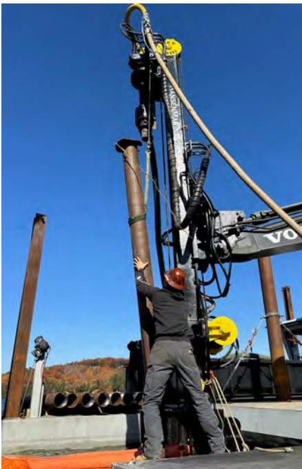
Drilling for the new support structure. Photo by Midge Eliassen.
