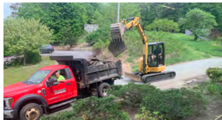
United Construction removing pavement to allow for the placement of stonework and vegetation.
