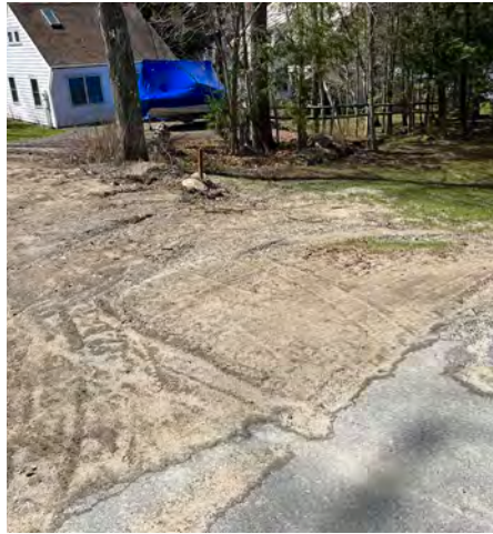
Before: Prior stormwater infrastructure implementation, sediment would wash downstream.
