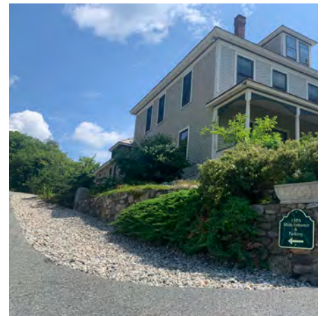
The finished project including stonework. LSPA will begin adding more vegetation upslope from the stone swale to further assist in stormwater runoff.
